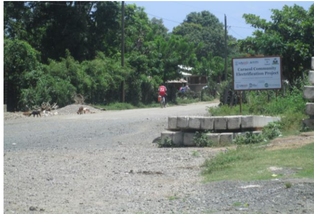
Unpaved road leading to Caracol village about 100 meters from the PIC gate. Caracol, Haiti © Gender Action 2013.
